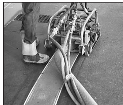
The JETTRAC™ Multicrawler System allows UHP Projects to utilize multiple automated robotic crawlers in conjunction with a powerful vacuum unit and 40,000 psi water to perform liner and coatings removal safely and efficiently.
