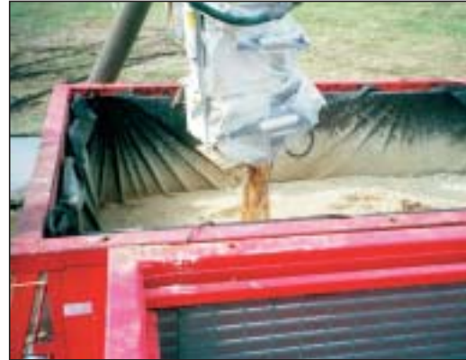
Effluent water and solids from JetTrac™ vacuum system.
