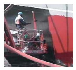
After each days cleaning, the cleaned area was primed using brush and rollers. The intermediate and final coats were also applied using brush and rollers. By using the covered vacuum cleaning method and brush and roller paint application there was no requirement to use drapes, tarps, booms or other equipment to protect the environmentally sensitive Elizabeth River or surrounding areas. During the two months that it took to complete this project there was zero spills or releases.
